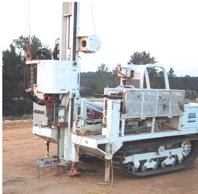
Figure 12 Small anchored drill-rig unit
